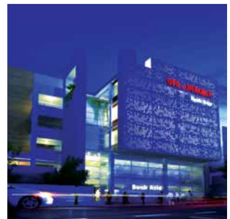
Outdoor Patient Department (OPD) building for Holy Family Red Crescent Medical College & Hospital
